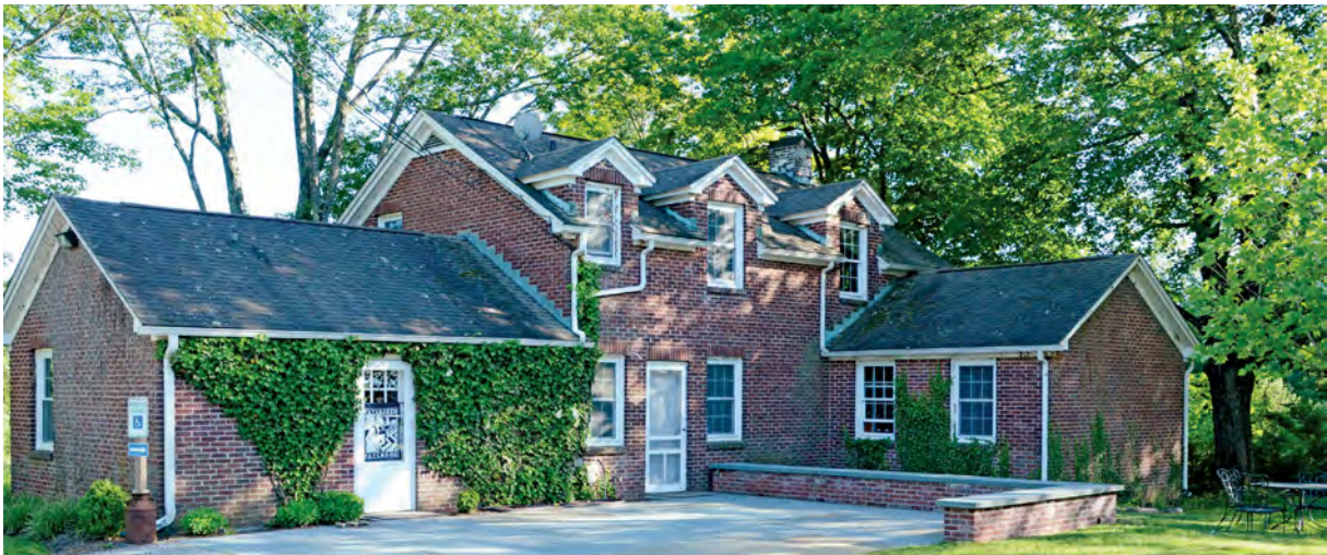
Betty Merck Science and Education Center. Houses staff, community meeting rooms and children's exploration room.
